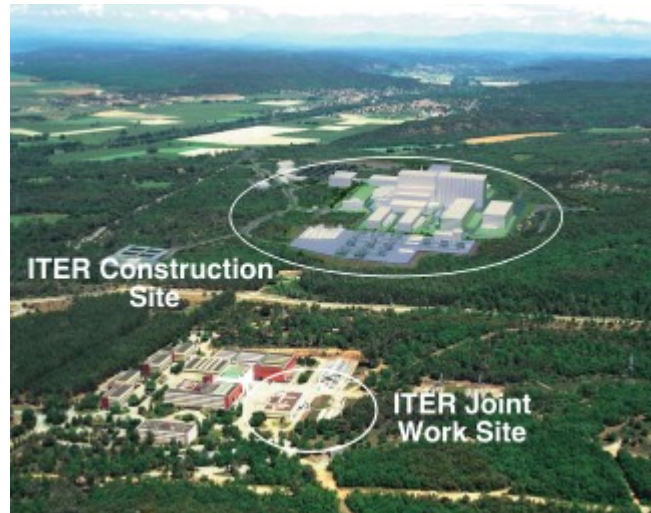
Figure 5: Impression of the ITER site (top). Below, the existing site of CEA is shown, which houses the Tore Supra fusion experiment.
